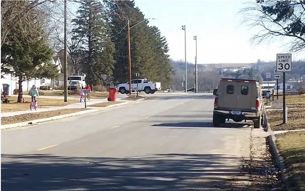
Photo of CSAH 2 in Elgin after 2017 construction
